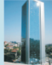
Polat Towers / İSTANBUL
